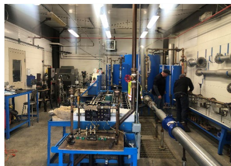
Water meter inspection. Photo Credit: OSA Staff
